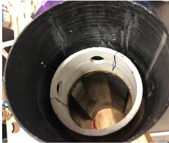
Figure 4-50 Centering ring and PVC extrusion
