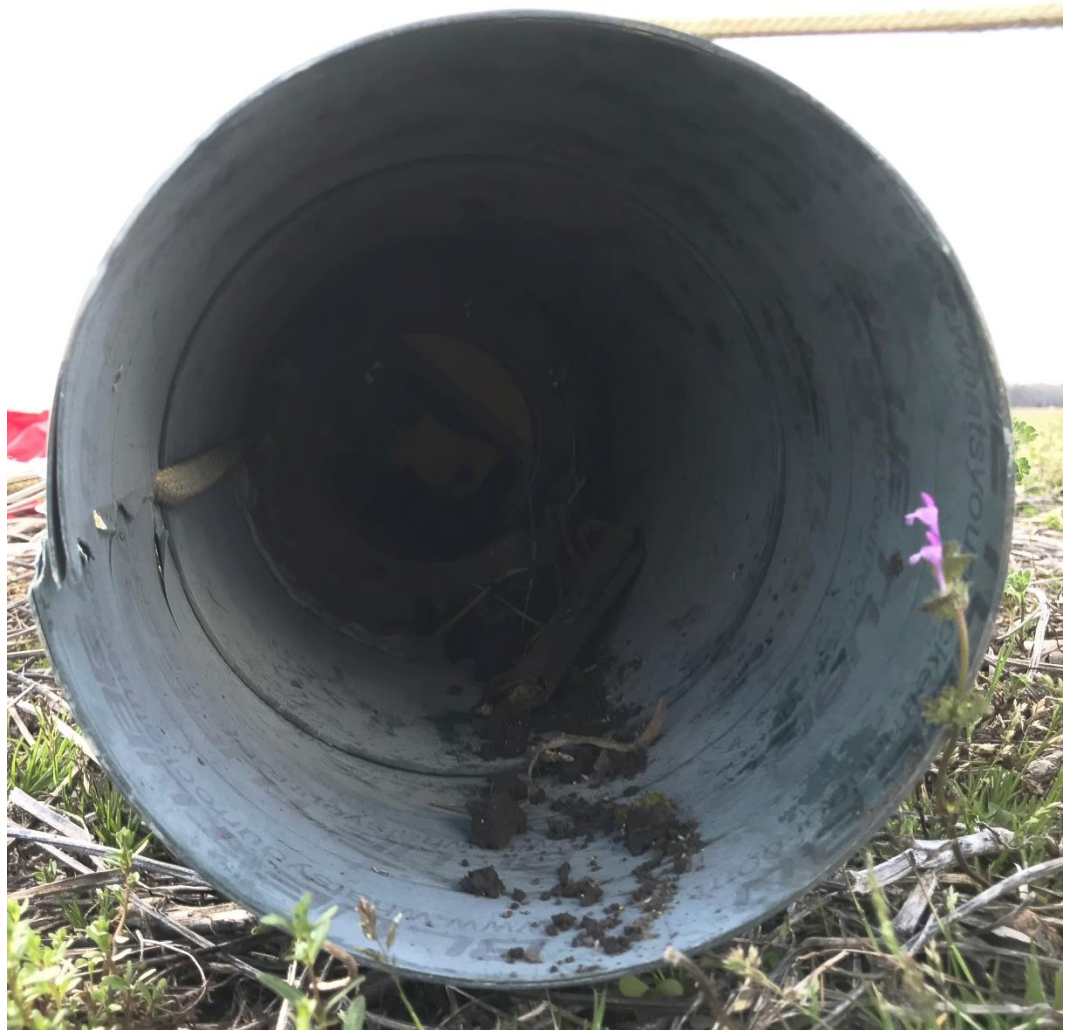
Figure 6-11: Midsection Zipper and Water Damage
